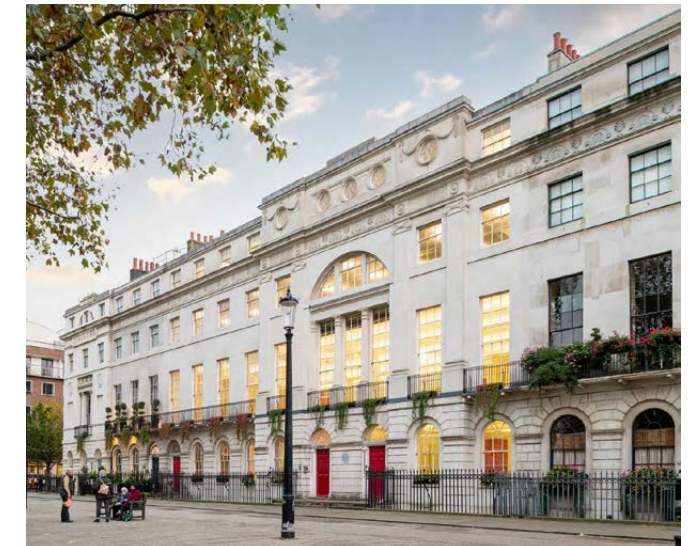
Boston House, 36-38 Fitzroy Square, W1
